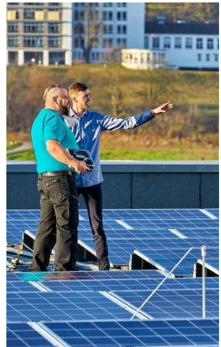
Uninterruptible energy generation
