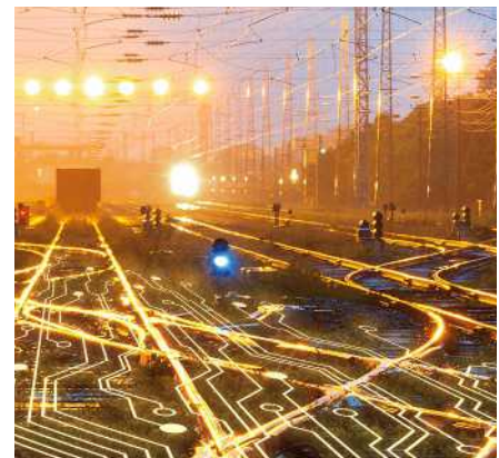
Modern railway infrastructure with surge protection
